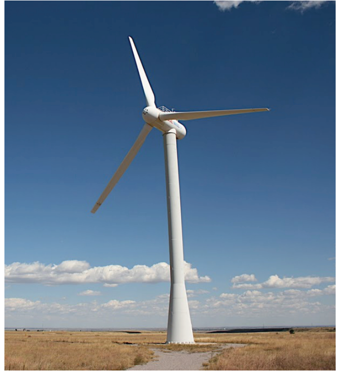
Fig. 1. The Controls Advanced Research Turbine (CART3) at the NWTC site at Golden, CO. Photo courtesy of Benjamin Sanderse from Energy Research Centre of the Netherlands.
