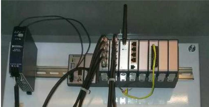
Figure A.1: The cRIO in the tower base used for CBM.
