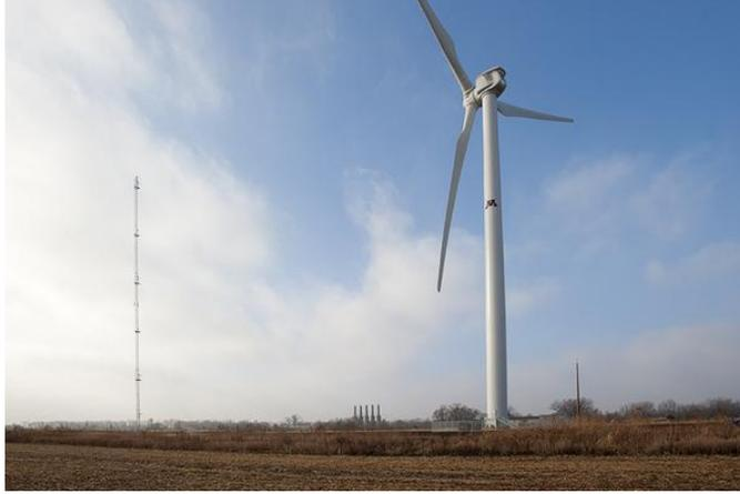
Figure 2.1: Clipper Liberty C96 2.5 MW wind turbine in University of Minnesota [2].
